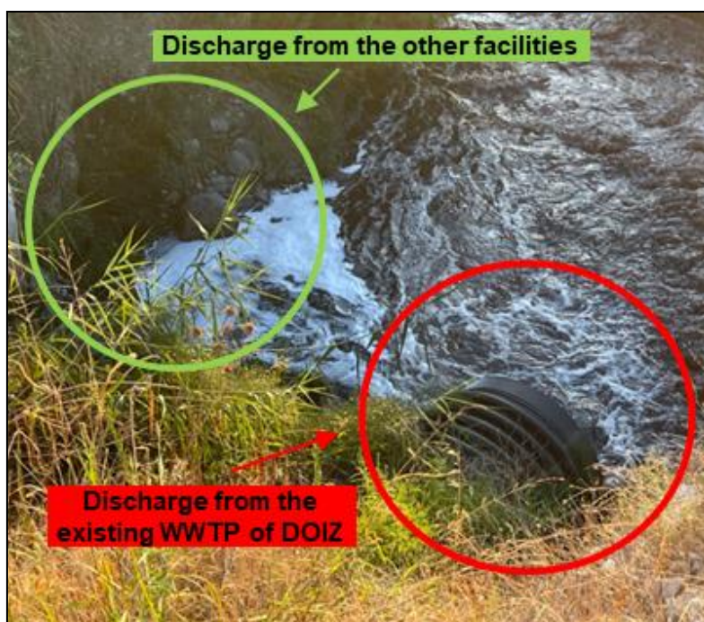
Figure 4.23 Photograph of Existing Discharge Point
