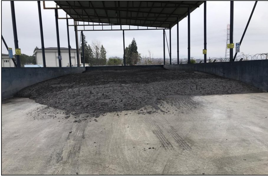
Figure 4.22 Temporary Storage Area for Sludge
