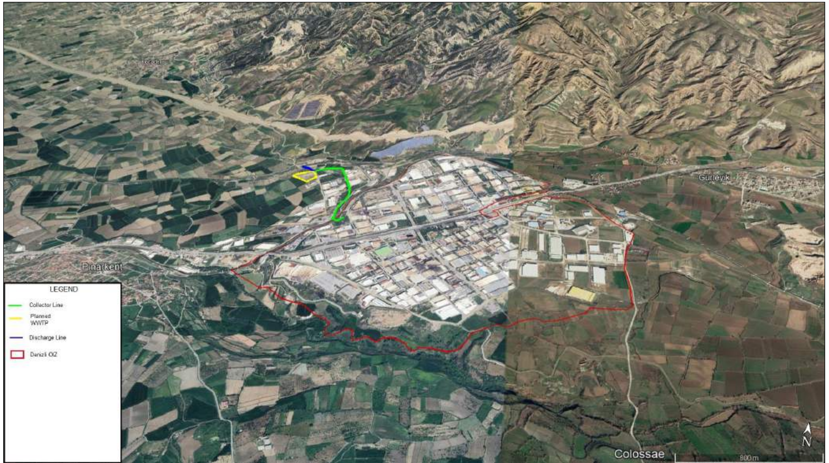
Figure 4.1 Satellite Image of the DOIZ (red polygon), Collector Line (green polyline), Planned WWTP (yellow polygon) and Discharge Line (blue polyline)
