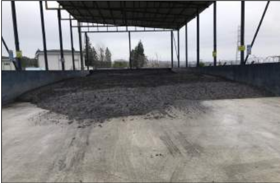
Figure 4.22 Temporary Storage Area for Sludge
