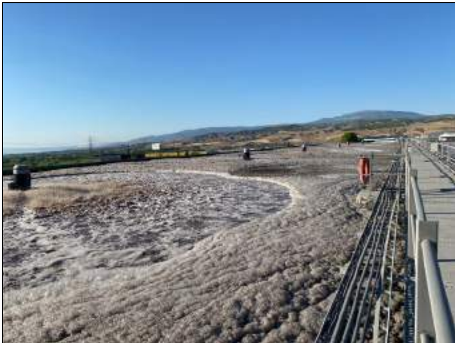
Figure 4.21 Photographs of Existing WWTP in DOIZ
