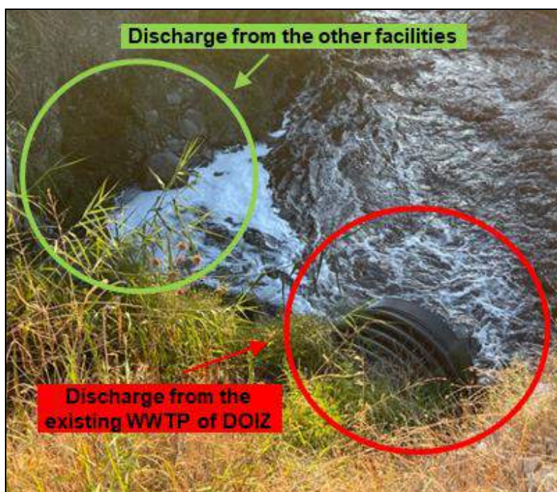
Figure 4.23 Photograph of Existing Discharge Point
